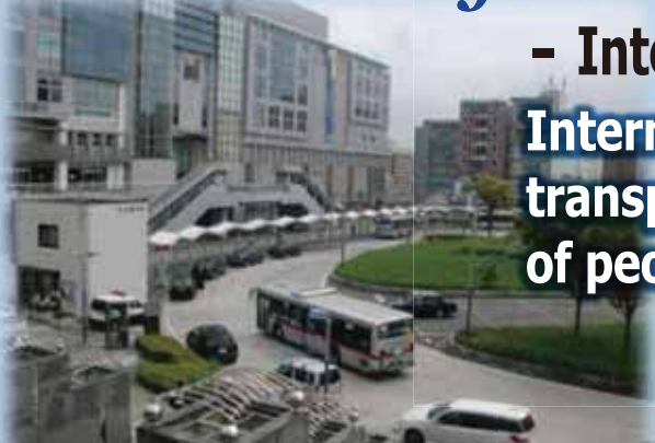
Intermodal Transfer Facility of Center Kita Station of Yokohama Municipal Subway (approx. 34,000 passengers/day)
