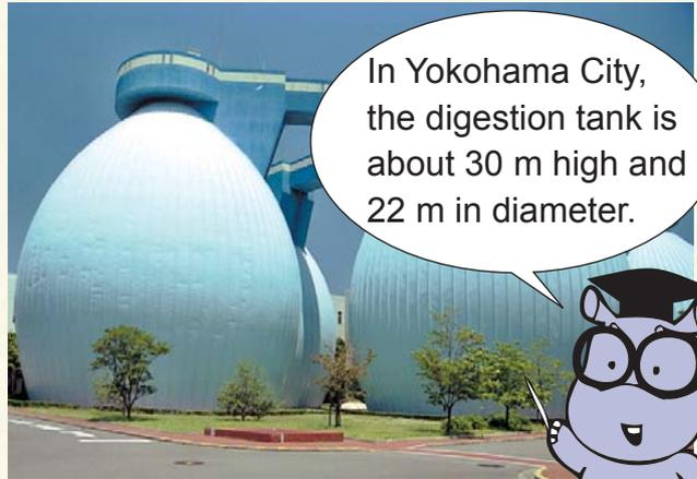
In Yokohama City, the digestion tank is about 30 m high and 22 m in diameter.
