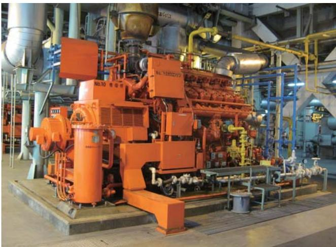
Gas generator for electricity generation running on digested gas
