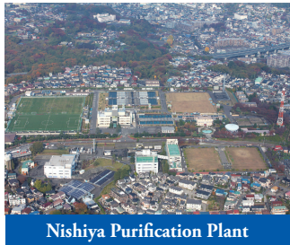
Nishiya Purification Plant
