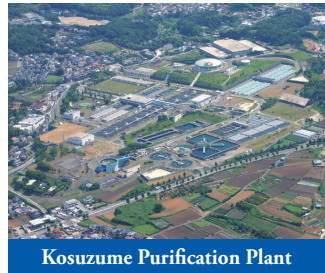
Kosuzume Purification Plant
