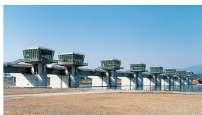
Sagami Ohzeki intake weir
