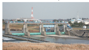
Samukawa intake weir
